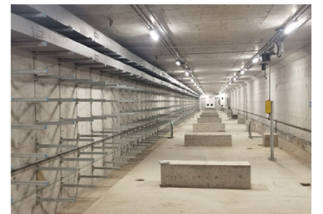
Utility tunnel construction 管廊施工
