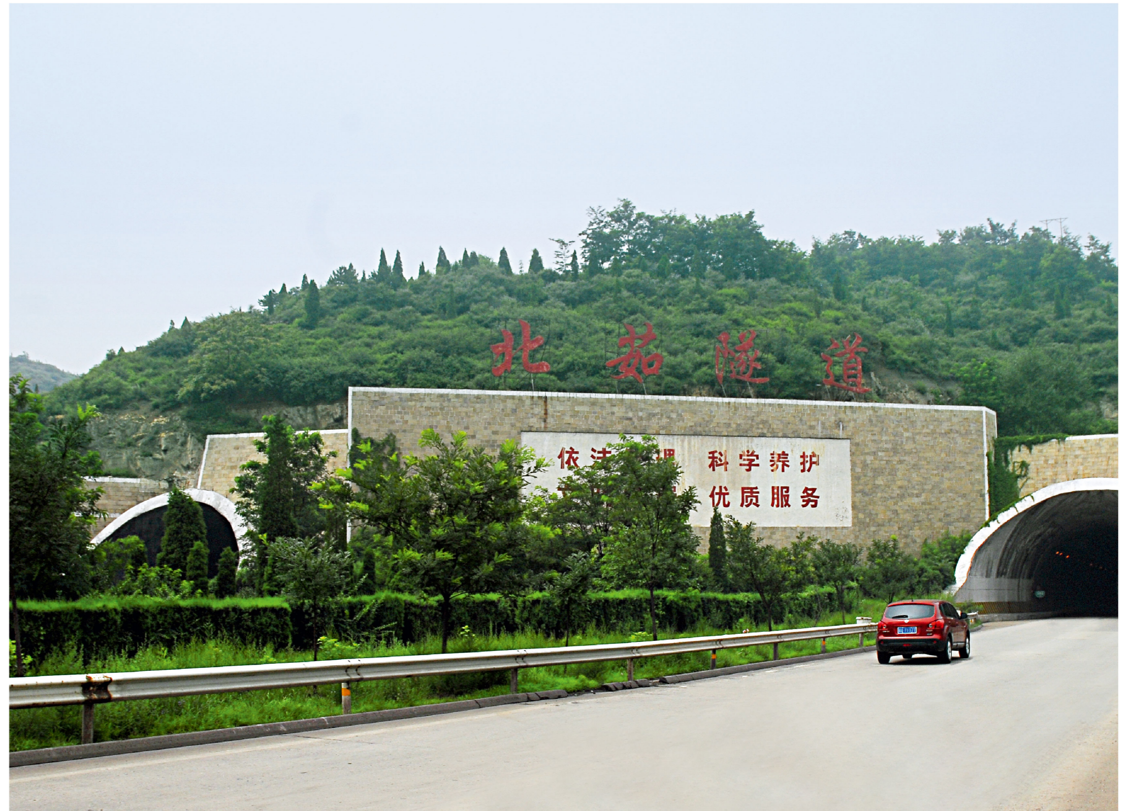
山西太旧高速公路北茹隧道工程 Beiru Tunnel Project of Taiyuan-Jiuguan Expressway in Shanxi
