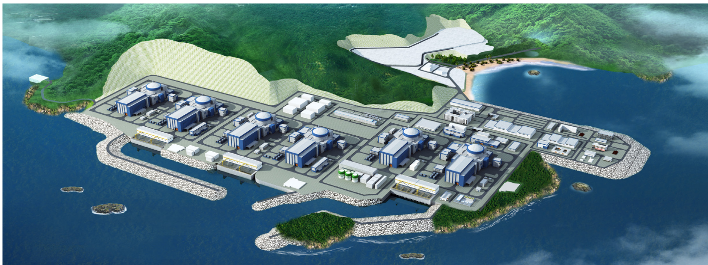
中广核三澳核电站一期北护岸、取水工程 North Revetment and Water Intake Engineering of San-ao Nuclear Power Plant (Phase I) of CGN
