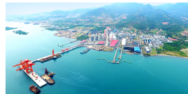
印尼海螺孔雀港项目配套码头工程 (国家优质工程奖) Supporting Specialized Wharf Engineering in Merak, Indonesia (Na- tional Quality Project Award)
