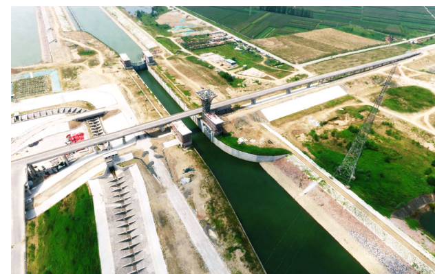
（世行贷款）汉江雅口航运枢纽船闸工程 Yakou Shipping Hub Ship Lock Project for Hanriver ( World Bank Loan )
