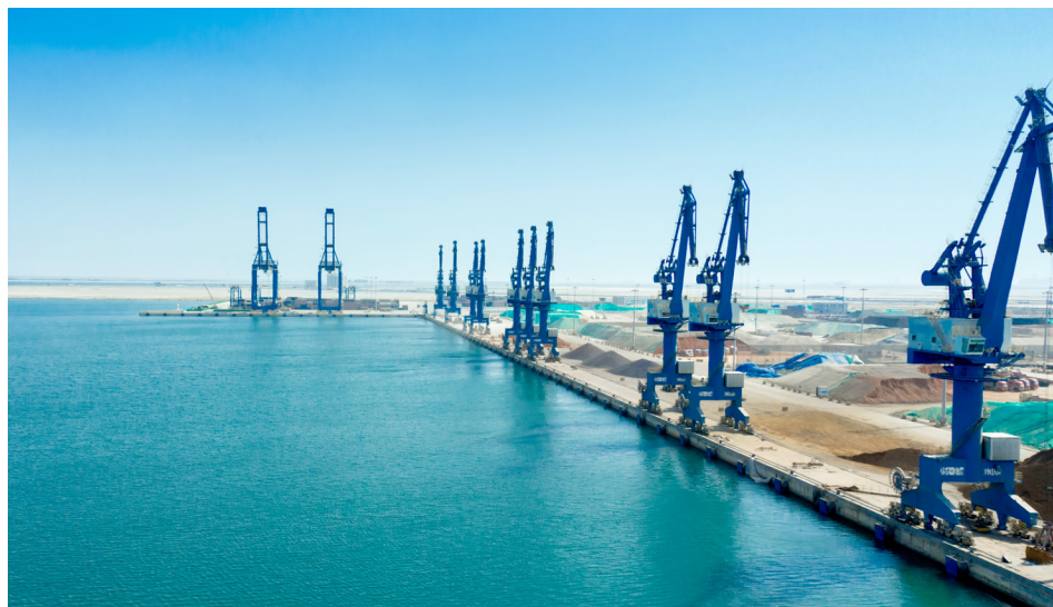
潍坊港中港区东作业区#18-#21泊位工程 (泰山杯) No.18 to No.21 Berths Construction Project of Port of Weifang ("Mount Tai Cup")
