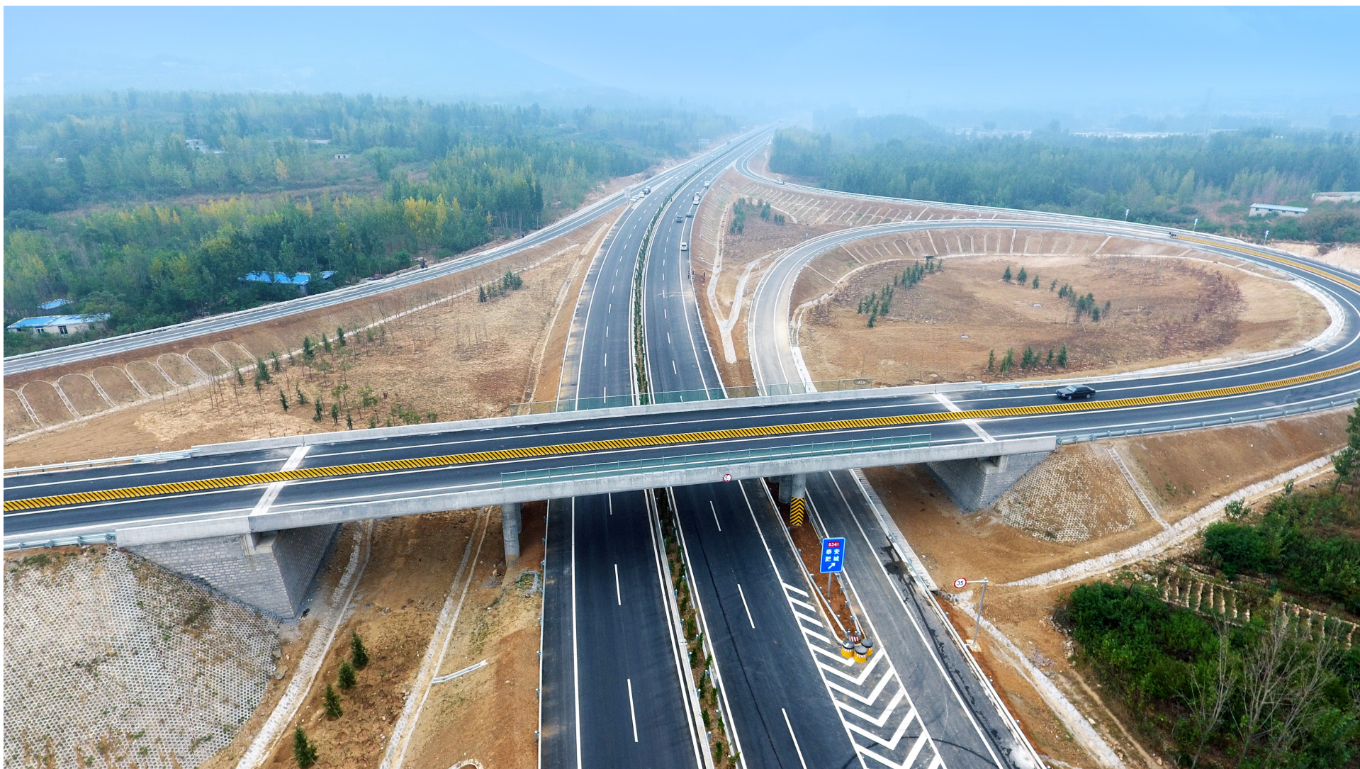
G104京福线界首至满庄段改建工程 G104 Jingfu Line Highway Renovation Project
