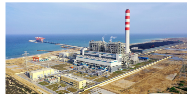
巴基斯坦中电胡布2×660MW燃煤发电工程 (国家优质工程金奖) Water Intake and Outlet Engineering of Hub Coal-fire Power Plant Project, Pakistan (National Quality Project Gold Award)
