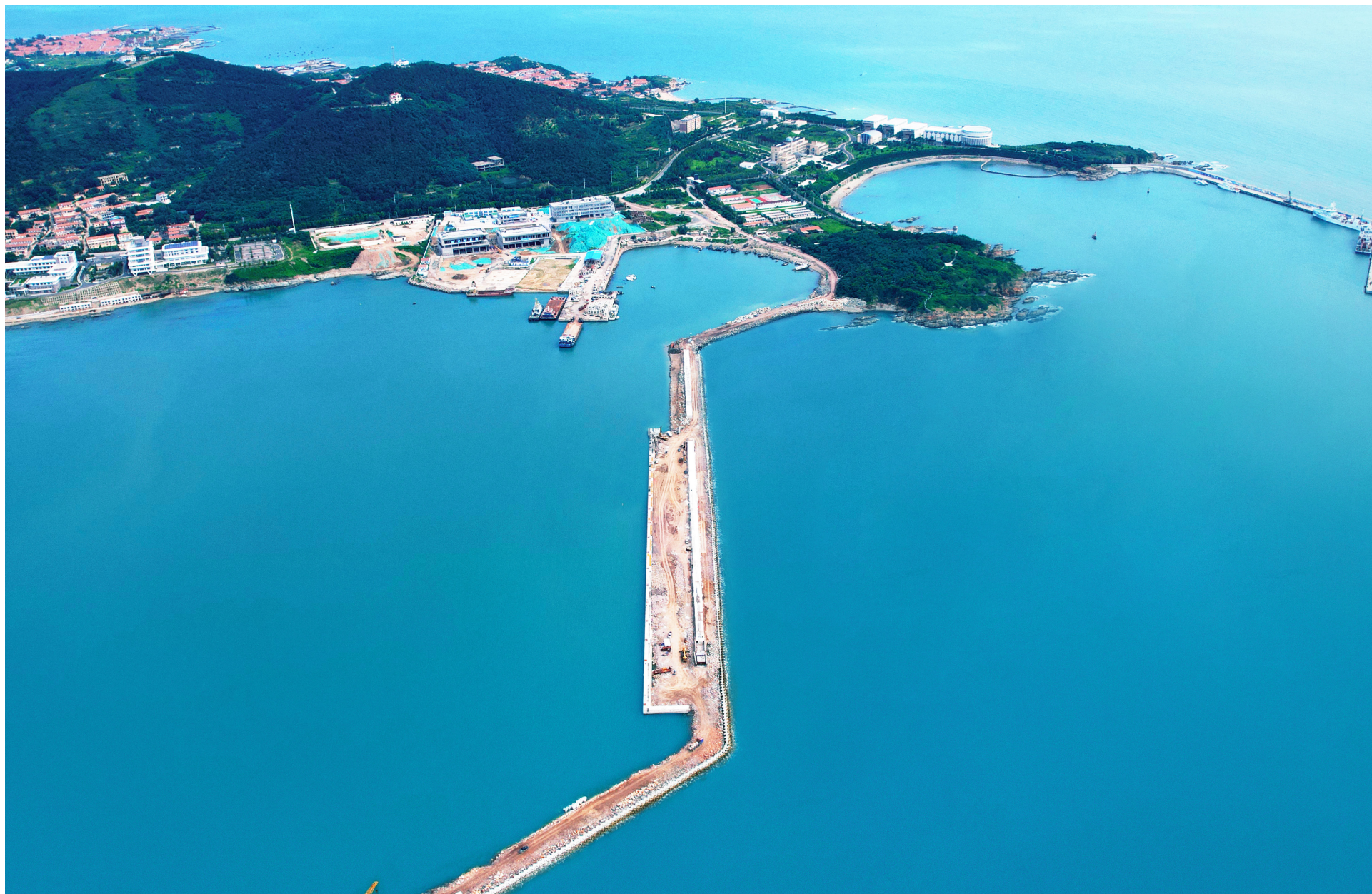
大洋钻探船码头建设工程 North Terminal Engineering of Natural Gas Hydrate Drilling Vessel Construction Project
