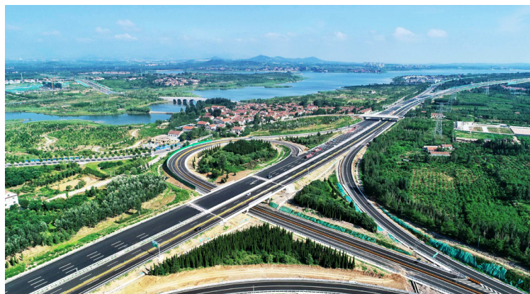
滨莱高速公路淄博西至莱芜段扩建工程 West Zibo to Laiwu Expressway Extension Project
