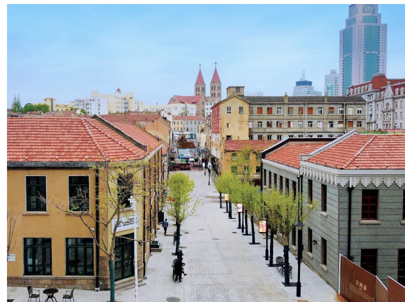
青岛市市北区“美丽街区示范区”工程 Demonstration Block in Shibei District of Tsingtao City
