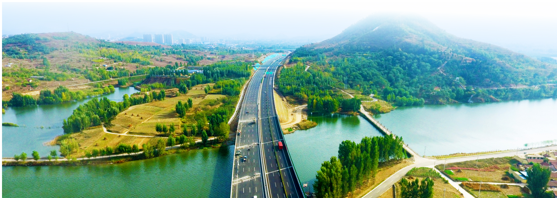
京沪高速公路莱芜至临沂（鲁苏界）段改扩建工程 Beijing-Shanghai Expressway Extension Project (Laiwu - Linyi Section)
