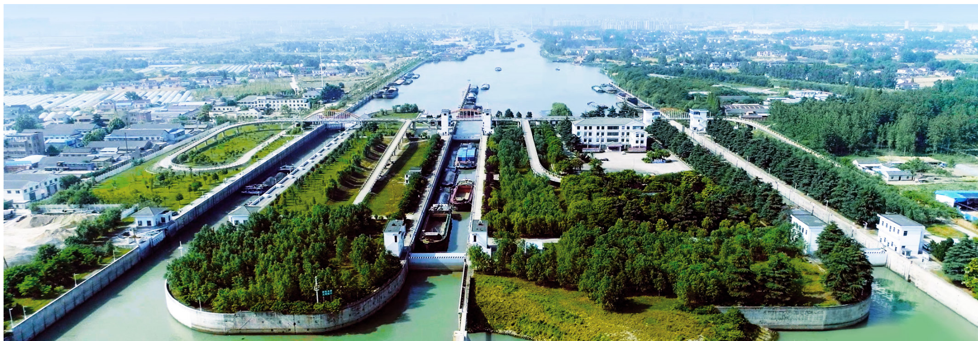
京杭运河扩容工程施桥三线船闸（国家优质工程奖） Shiqiao Third-line Ship Lock Project of Beijing-Hangzhou Canal ( National Quality Project Award )
