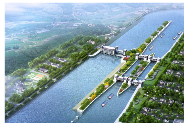
魏村枢纽扩容改建工程 Weicun Ship Lock Expansion Project
