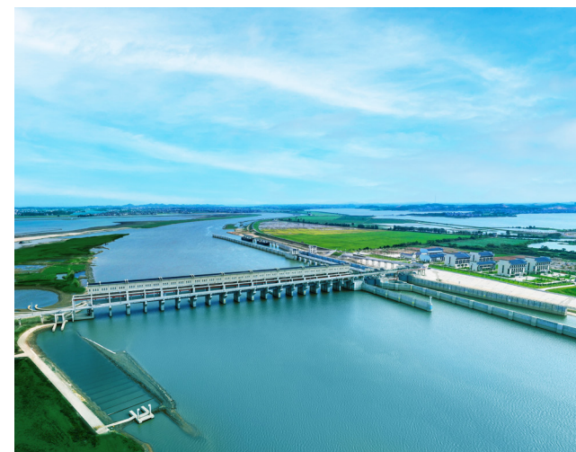
江西信江双港航运枢纽主体工程 Shuang-gang Shipping Hub Project, Jiangxi Province
