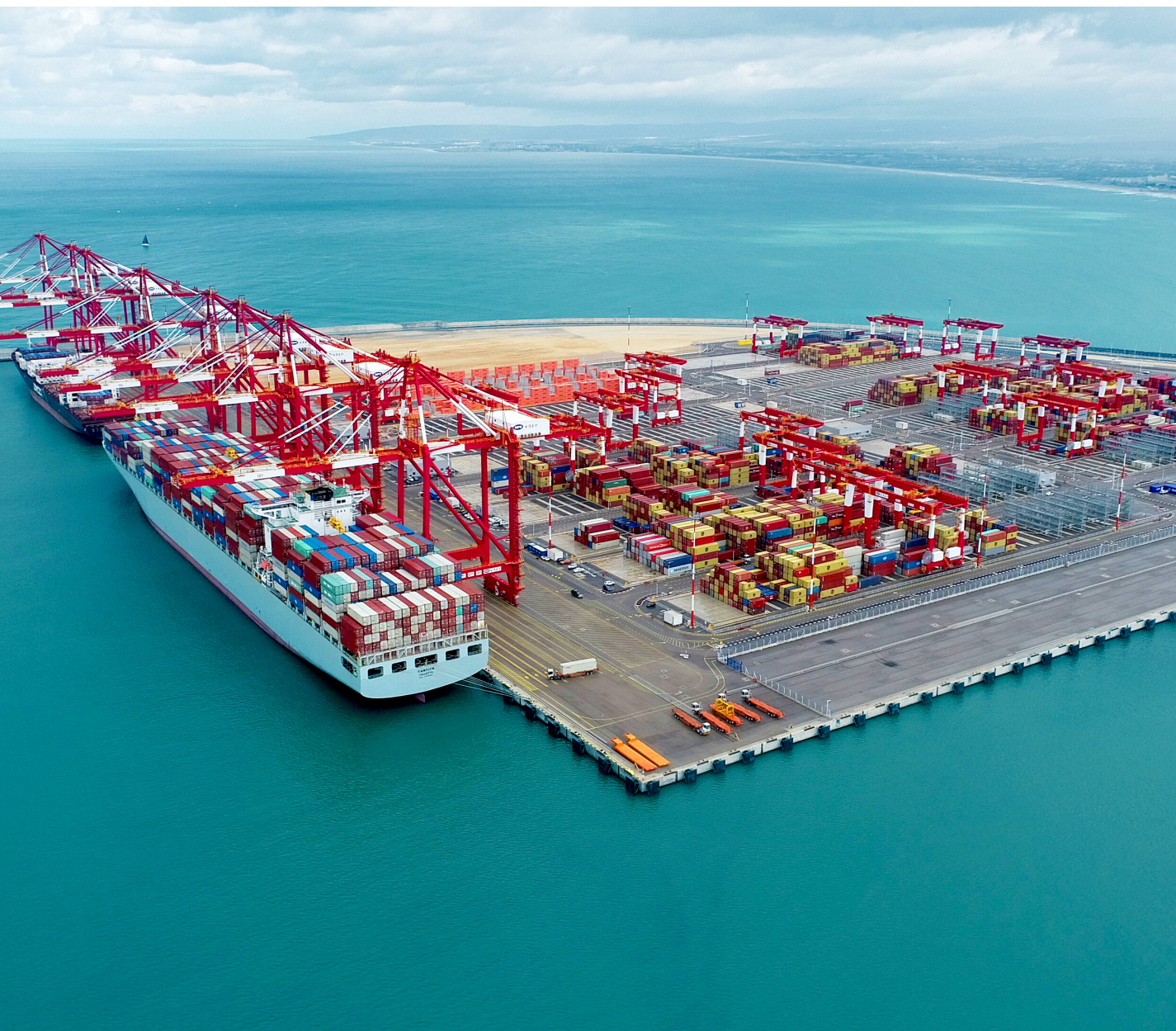
以色列海法 BAYPORT 港口工程 (EPC) (鲁班奖) The Operation and Maintenance of the Bayport Terminal in Israel (EPC) (The Luban Prize)
