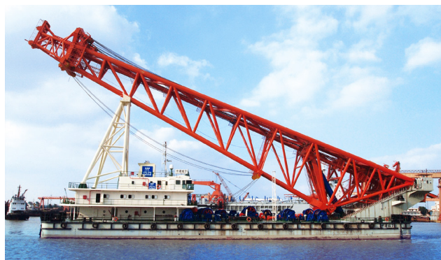
中建桩7 (桩架高110米) No.7 Pile Driving Barge
