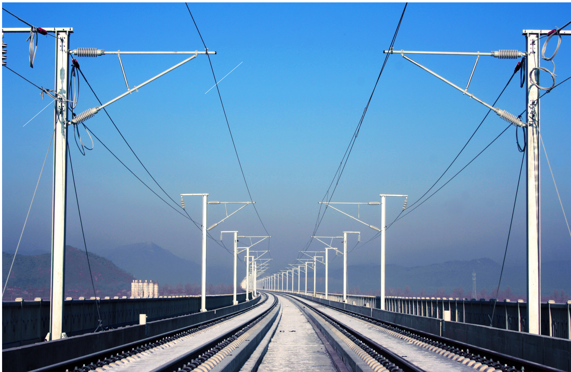
辽宁省沈阳至丹东客运专线工程 Shenyang – Dandong High-speed Railway Project in Liaoning Province
