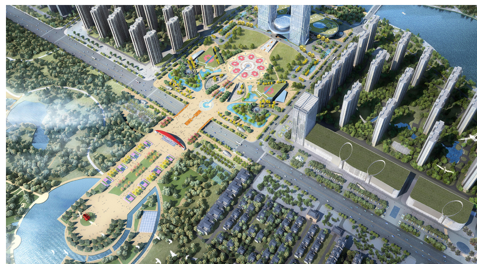
曹州牡丹园东广场防空专业队及人员掩蔽工程 Underground Parking Lot ( Air Defense Shelter ) in Caozhou City
