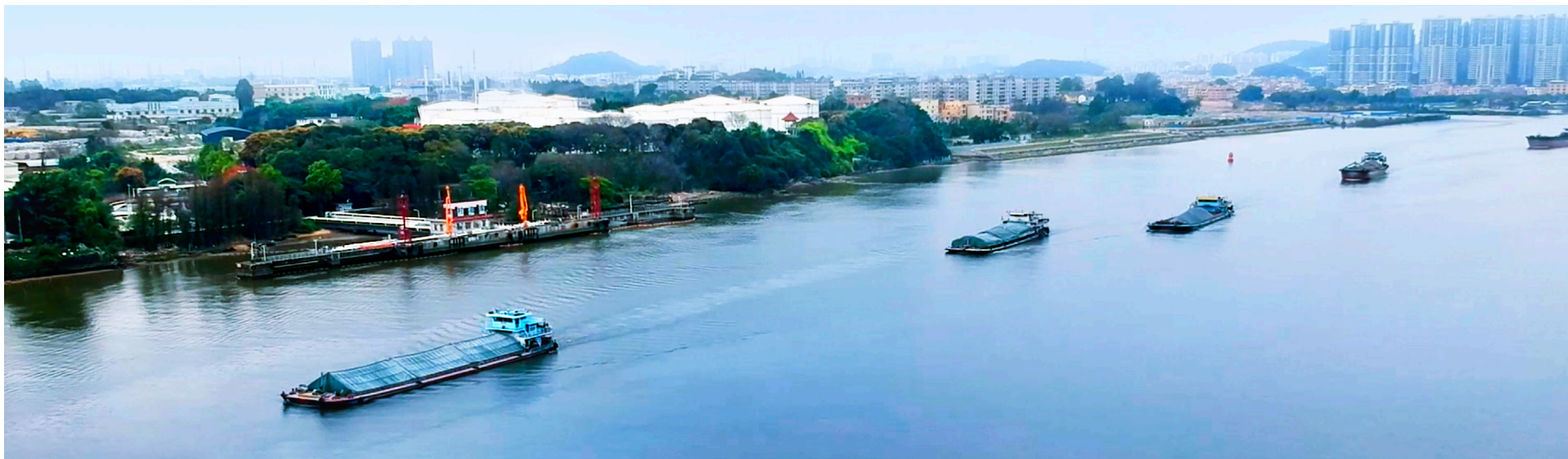
秦淮河（溧水石臼湖-江宁彭福段）航道整治工程 Waterway Regulation Project of Qin Huai River
