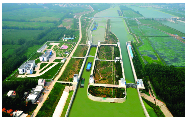
京杭运河台儿庄复线船闸（泰山杯） Taierzhuang Double Track Shiplock on the Beijing Hangzhou Canal ( Taishan Cup )
