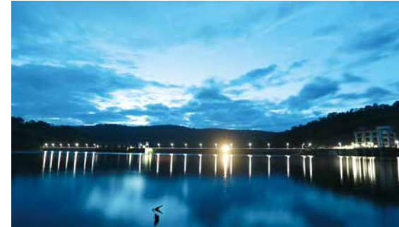
甘再电站大坝清晨
